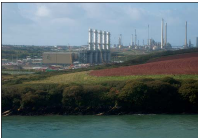
The new gas-fired power station at Pembroke, and behind it the Valero oil refinery Photo: Gordon James
